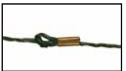
If making a repair over a vertical stay, weave the connecting twine over and under the black plastic joint.
