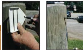
2. Install End Post Attaching Buckle (ribs away from end post). Use Bending Tool to accurately shape rail.
