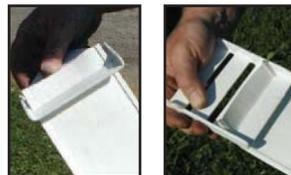
2. Use the buckle as a tool to bend the end over as shown. Always bend towards the BACK of the rail. After removing the buckle you should have an approximate 2" bend. Repeat process on second rail end for joining.
