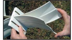
2. Use the Bending Tool to accurately shape the rail, creating an "M" as shown in this inset photo.
